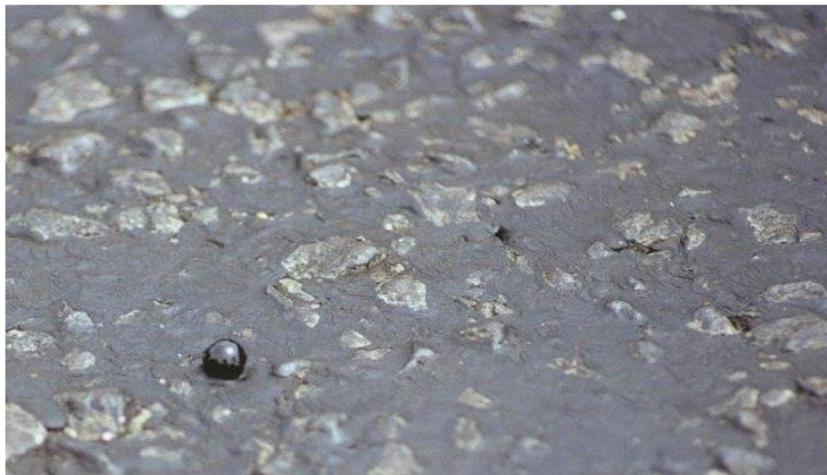
**Photo of bitumen bubble.** Note also vent holes from former bubbles now partially closed by traffic.
